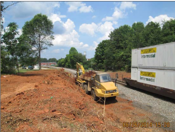
P-5206 Reid to N. Kannapolis - Grubbing
