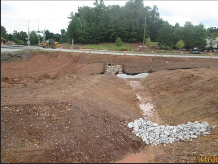
P-5201 Morrisville Parkway grade crossing
