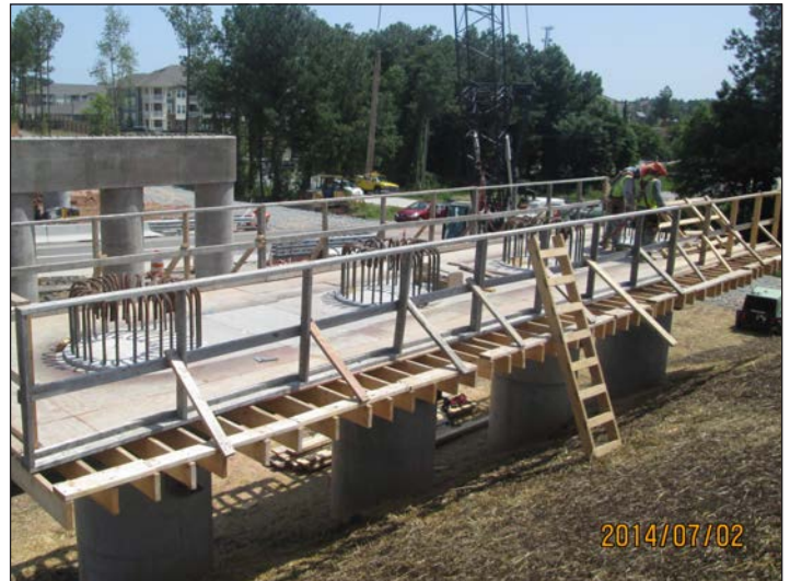
U-4716 RR Bridge over Hopson Road
