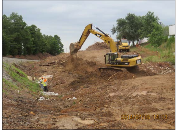
P-5201 Morrisville Parkway, east approach to bridge
