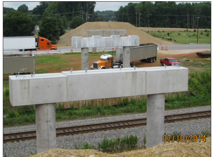
P-5206 Peeler Road Bridge Construction
