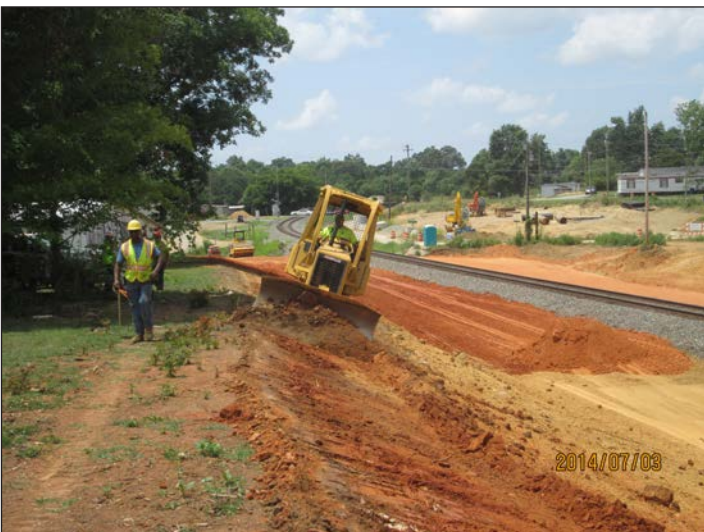
P-5205 Graham to Haw River Grading
