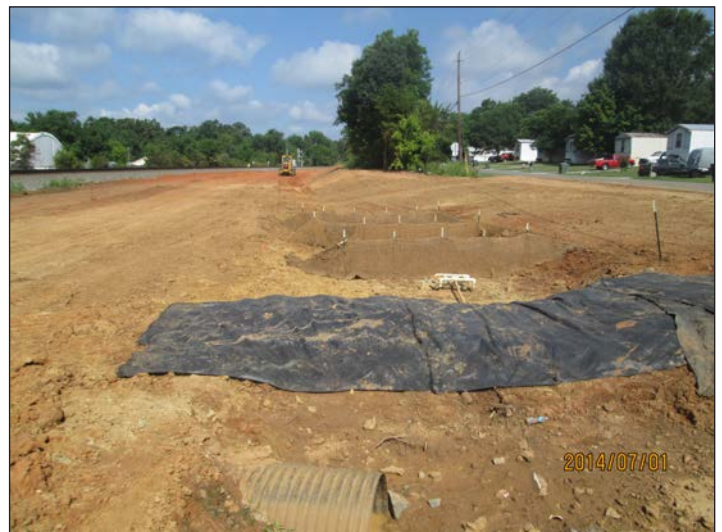
P-5205 Graham to Haw River Erosion Control
