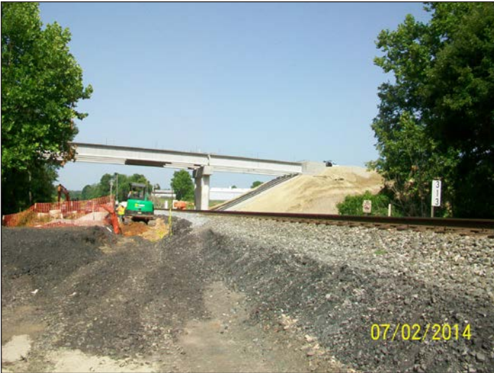
C-4901 Bowers to Lake - Turner Road Bridge
