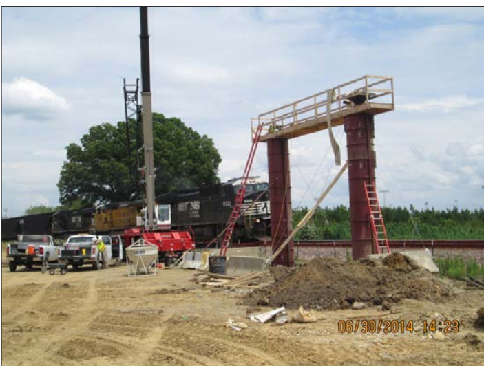
P-5208 Haydock to Junker - Roberta Road overpass
