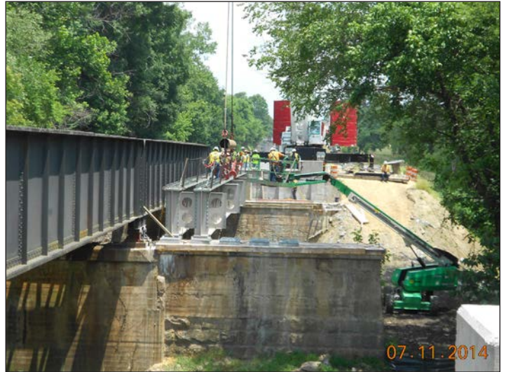
C-4901 Bowers to Lake - Hamby Creek Bridge
